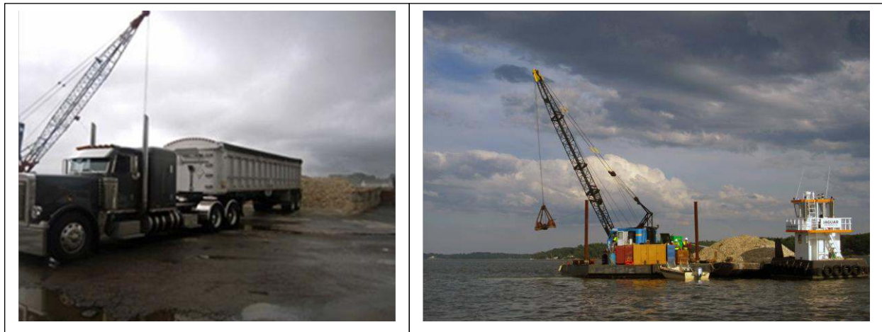
Fig. 3. Shell delivery by truck at Granite State Minerals, and reef shell base construction by Riverside and Pickering Marine.
